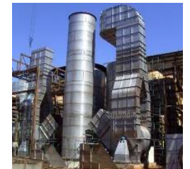
Carbon steel substitution
